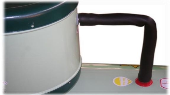
Picture 1.21 Install the pipe isolation.
