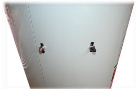
Picture 1.12 Thread protecting rubbers are being removed
