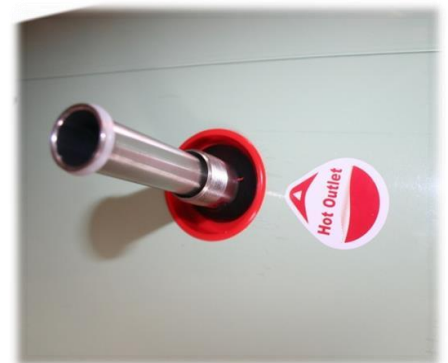
Picture 1.24 Install a stainless steel pipe in the hot water outlet.
