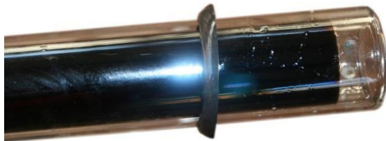
Picture 1.18 Fill the tube with water, install the rubber and lubricate the open end of the tube
