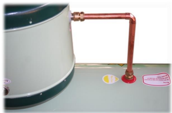
Picture 1.20 Connect the geyser overflow to the reservoir
